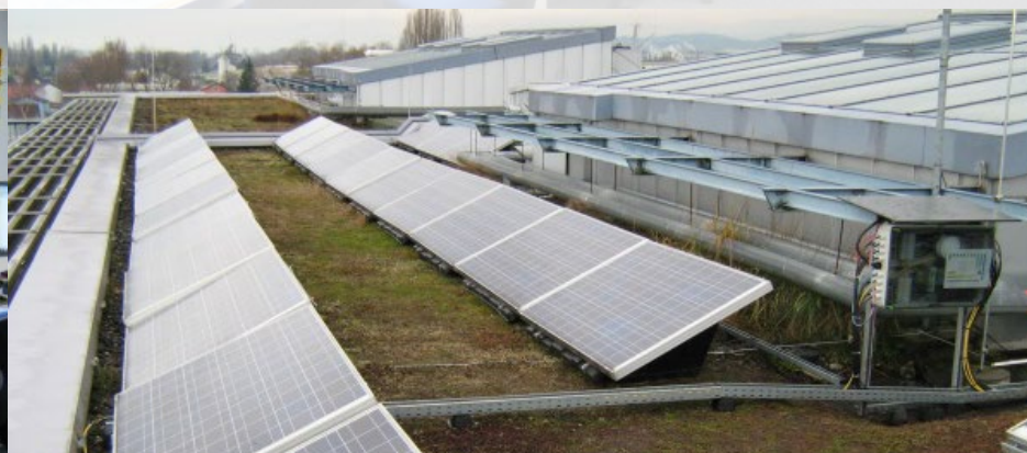
PV Installation 9 kWp
