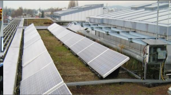
PV INSTALLATION 9 KWP
