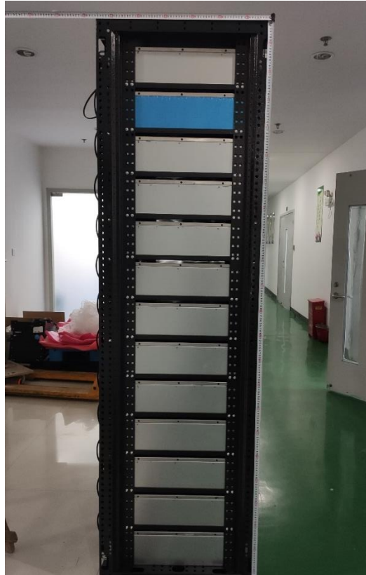
Figure 7 Battery System (Side view for 25 modules)
