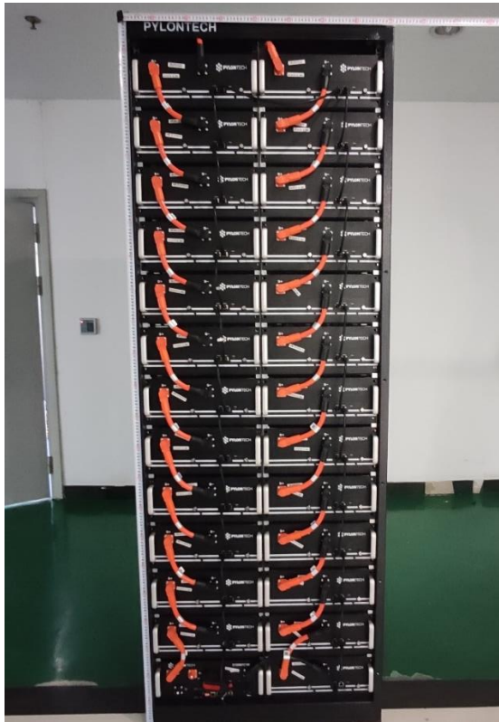
Figure 5 Battery System (Front view for 25 modules)
